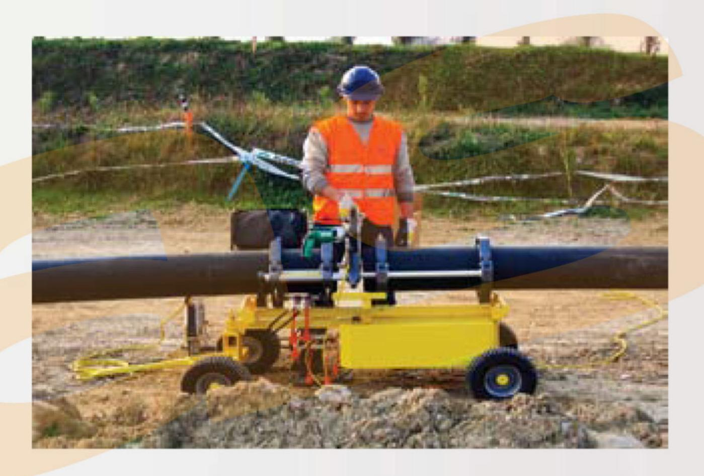
Clamps are used correctly to ensure that nomovement of the joint can take place during the heating and cooling cycle.
